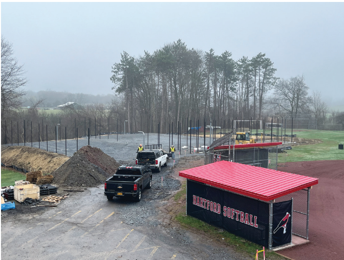
The image shows the outline of the batting cage and courts. The area is being prepared for the asphalt.
