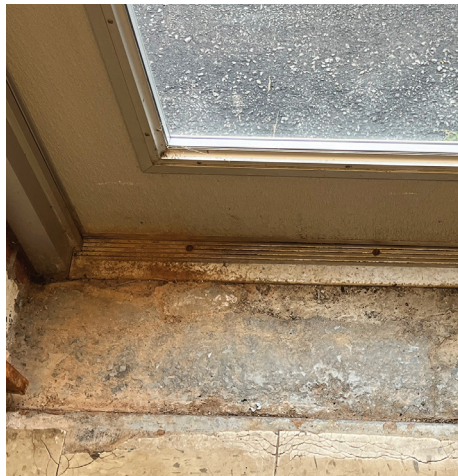
Deteriorated flooring by the Art Room entrance from the back parking lot.
